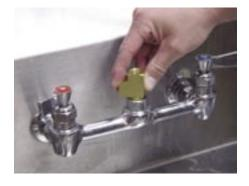
Step 4 Screw in hose fitting and reatttach prewash sprayer.
