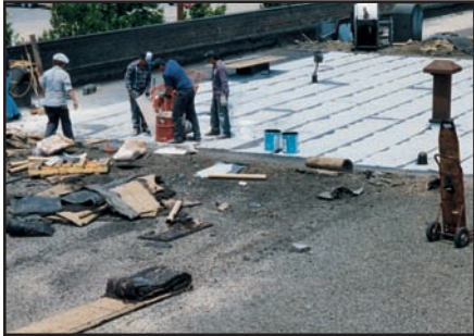
Unnecessary Roof Repair
